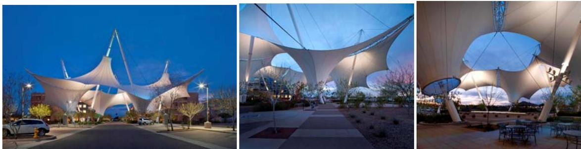
Besides the membrane providing about 80% shade, in the evening the lighting of the membrane is done with both LED lighting in a blue color on the A-frames and white HID lighting on the fabric surfaces.
