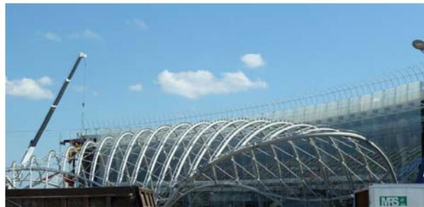
Steel was completely prefabricated off site and each piece was tested to fit in the shop before shipping to site which allowed for a clean and tight fit on site. Foil pillow extrusions were attached and the prefabricated foil cushions were installed and pressurized. LED lighting was then installed and tested for color range and connections.
